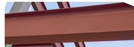
ST - Painted steel in a heritage red type colour
